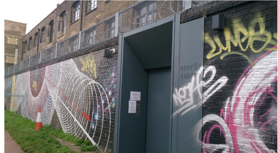
East London Office - Main Entrance
